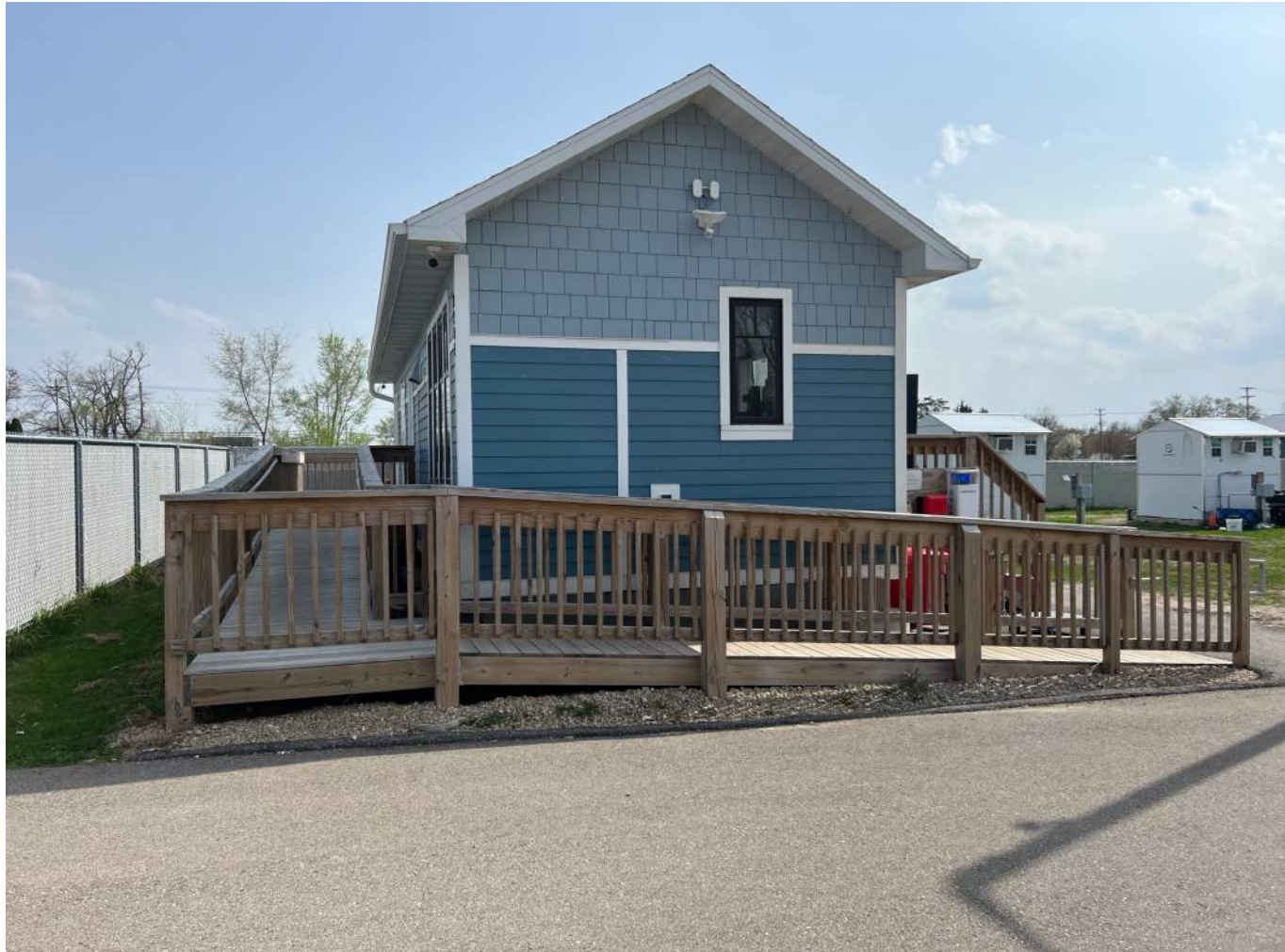
EXISTING BATHROOM/OFFICE BUILDING
