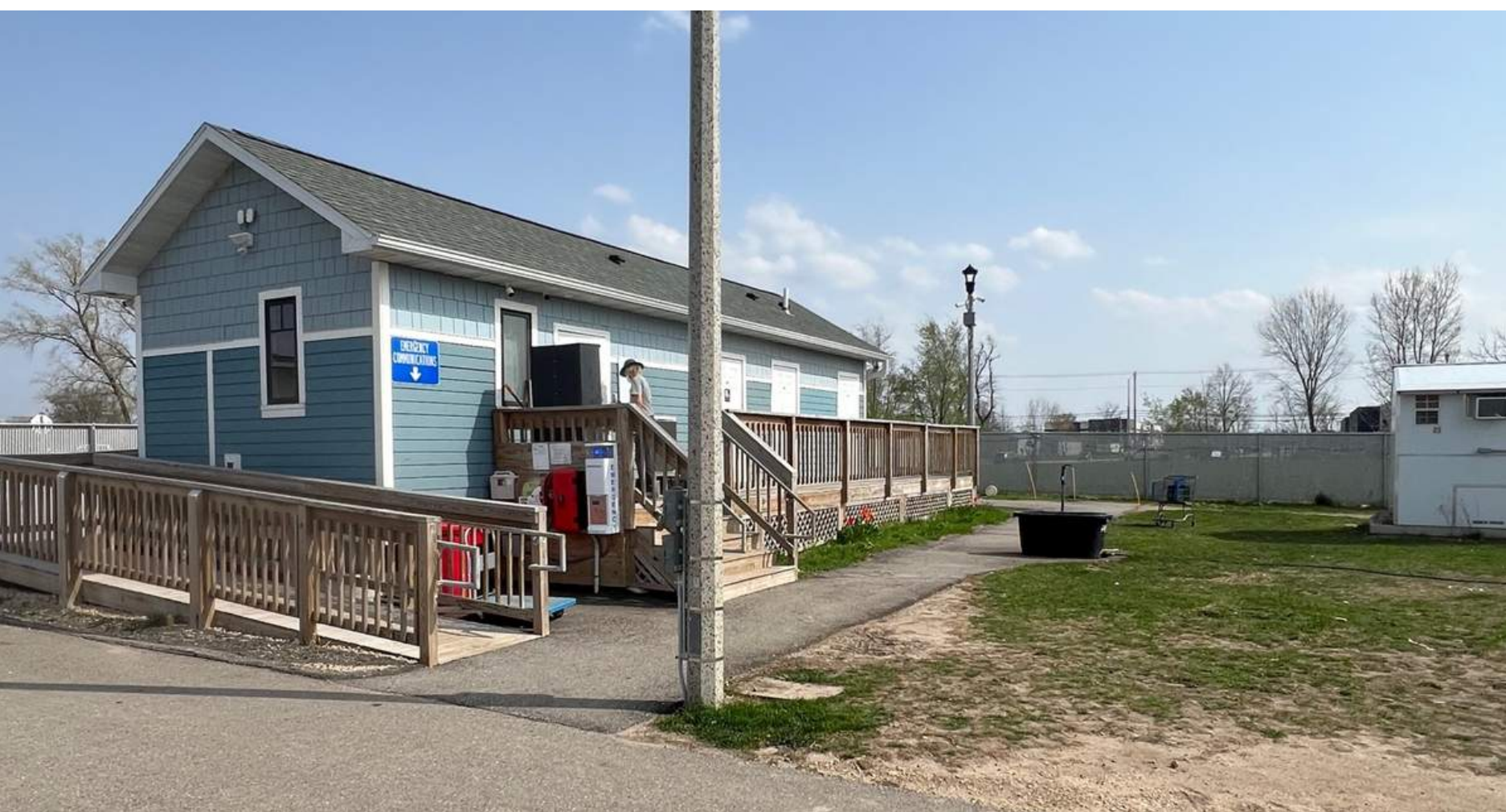
EXISTING BATHROOM/OFFICE BUILDING
