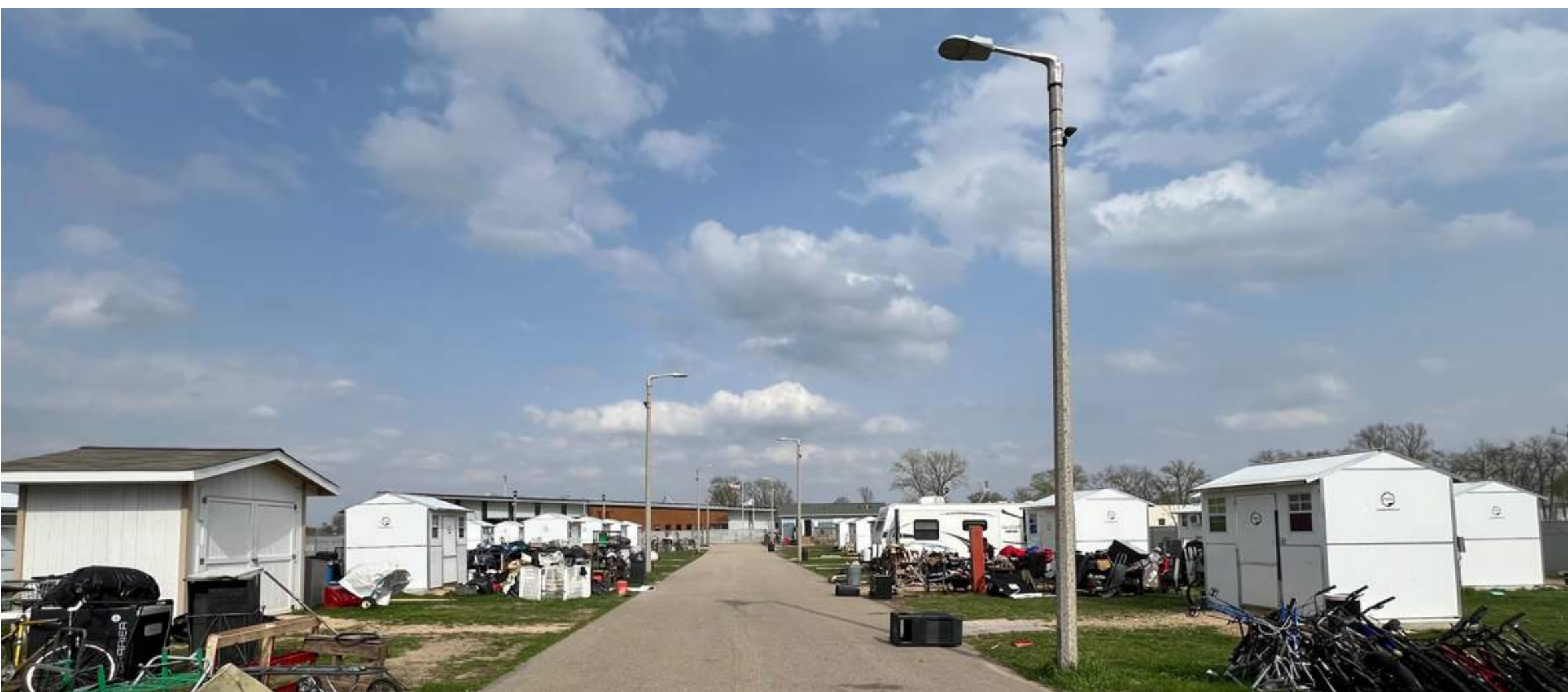
FIRE LANE LOOKING EAST
